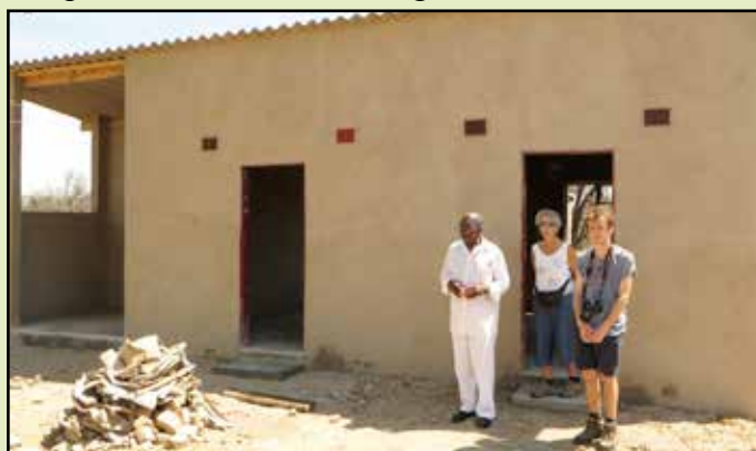
Nearly completed maternity waiting rooms
