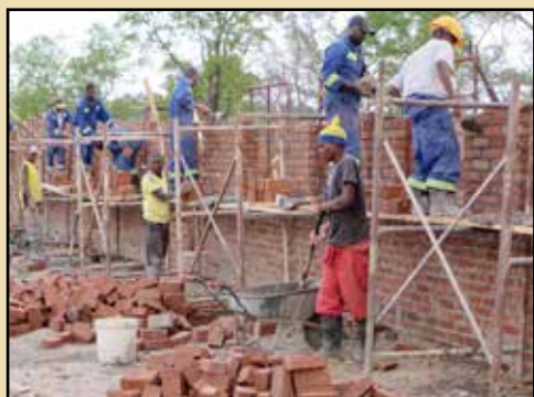
Impressive bricklaying at Chiwodza secondary school
